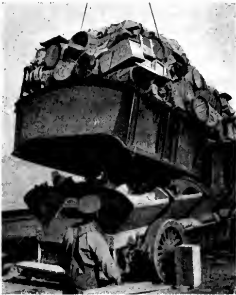
Unloading at docks by electric hoist.
